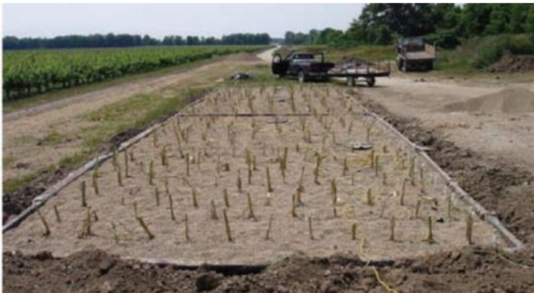
Figure 4-9 : Typical Constructed Wetland (Still under construction)
